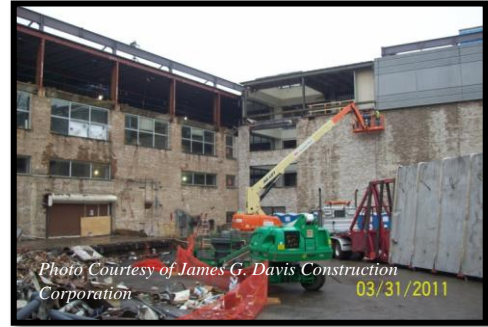
Figure 2 | Demolition of Existing Parapet for Perimeter of Main Building
